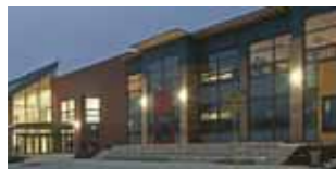
Schulkomplex Roodt-Syre, Lx School Complex, Luxemburg
